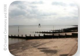
**Revetments** – Wooden walls made of water-resistant wood. Blocks waves and stops sand being washed away. Cheap and easy to build. Very Ugly.
