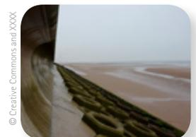
**Beachfeed** – Tonnes of sand is dropped on a coast to form a 'fake-beach'. Beaches look nice and can be used by tourists. Sand is cheap. It needs constant maintenance as much of the sand gets washed away and needs replacing.
